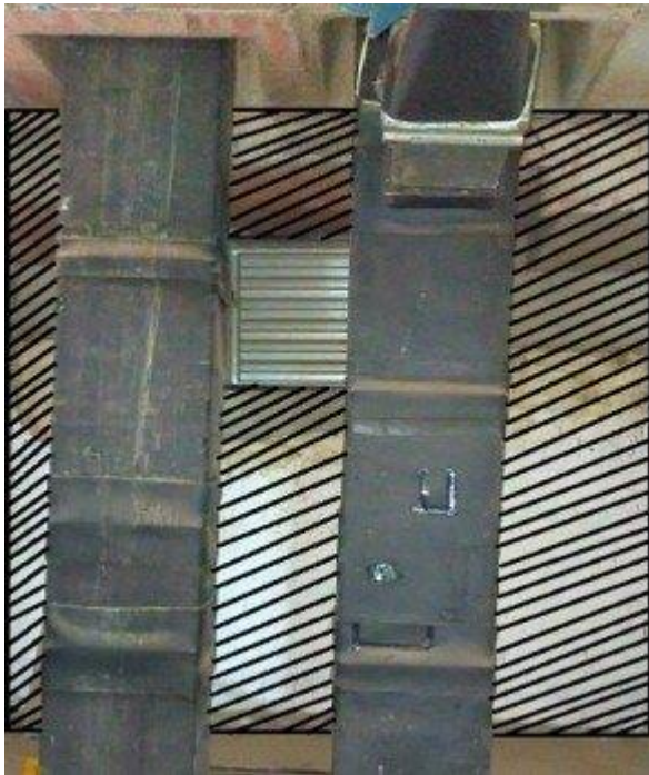
Part wall demolished for blower unit
